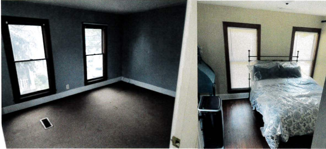
Bedroom 2 – removed carpet and repaired/refinished Heart Pine floor
